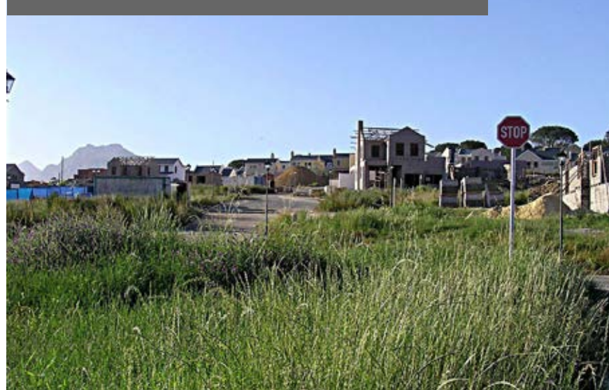
November 2004 - A general view of the building activities.
