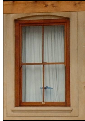
Figure 10: Vertically proportioned window with plastered window sill and simple plaster-band forming a flat arch above the window.
