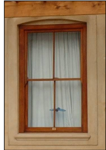
Figure 10: Vertically proportioned window with plastered windowsill and simple plaster-band forming a flat arch above the window.
